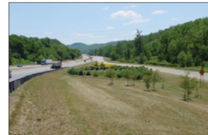
Online Bioretention Area
